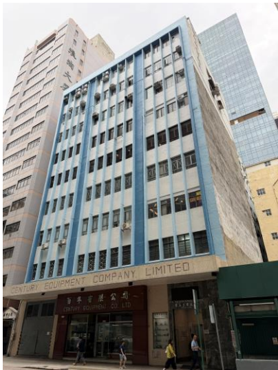
3 Yick Tai Industrial Building
