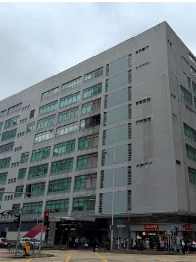
4 Hong Kong Spinner Industrial Centre Phase I & II
