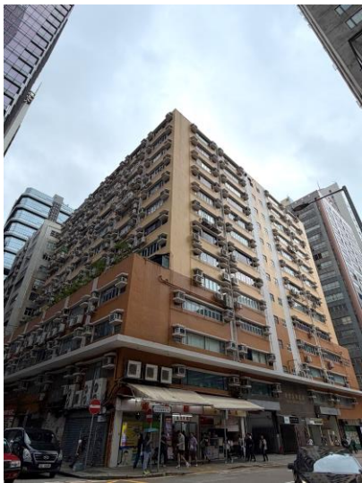
6 Wing Kut Industrial Building
